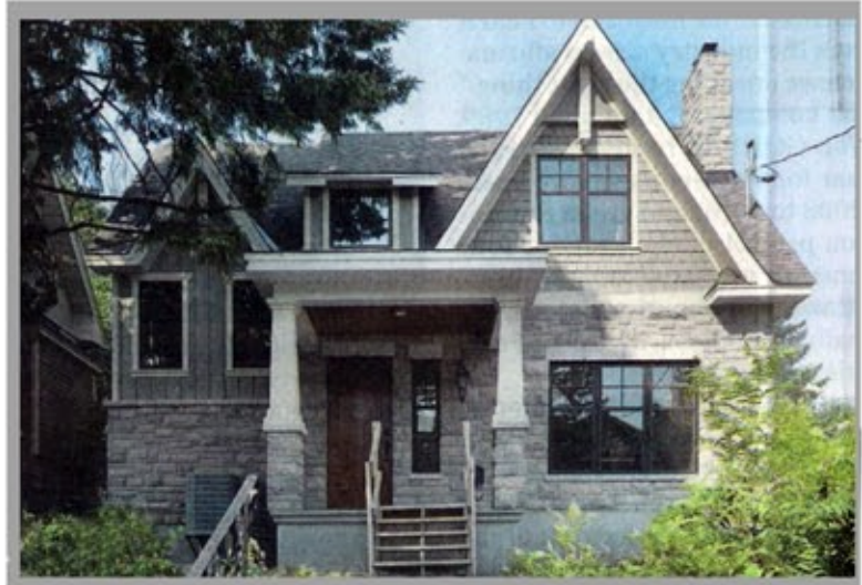
Amsted Design-Build and Chuck Mills Residential Design & Development won for renovation, $500,000 to $749,999. (The steps are temporary.)
